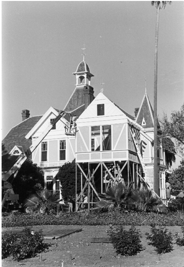
A western view of the faux gable during construction.
